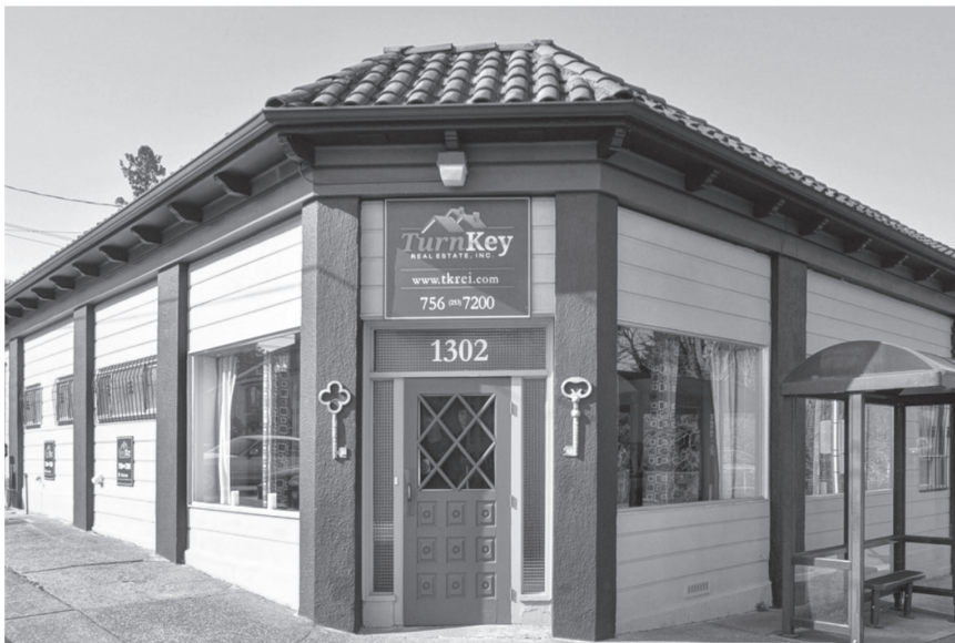
1302 N I Street, Tacoma, WA 98403
